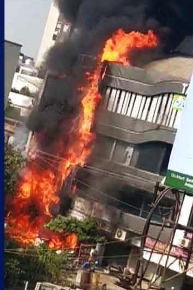
Heat from initial fires ignited banner and the cable duct, and travelled to the fourth floor (other floors relatively unaffected)
