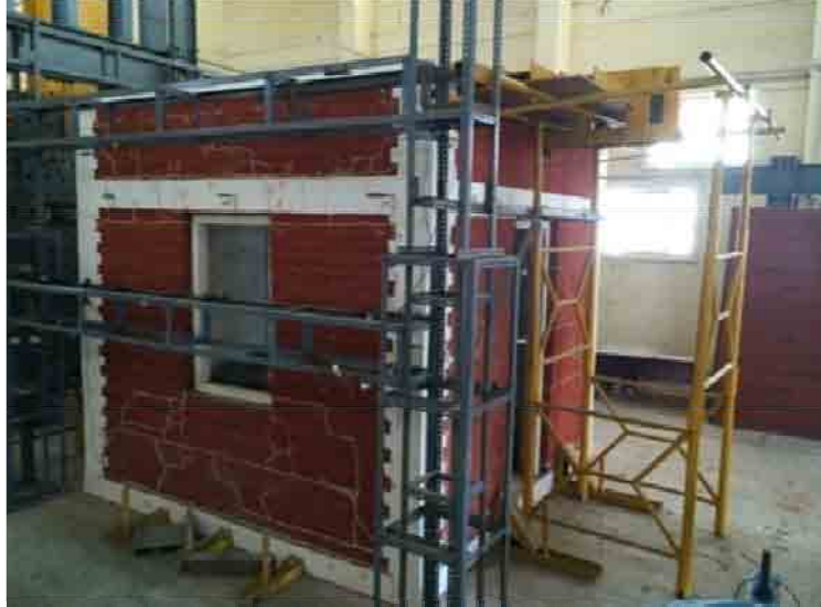
Cracks in CM building Model
