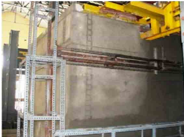
Plastering and Curing
