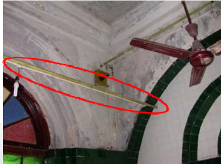
Tie-rods placed in both directions
