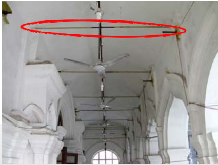
Tie-rods placed in both directions
