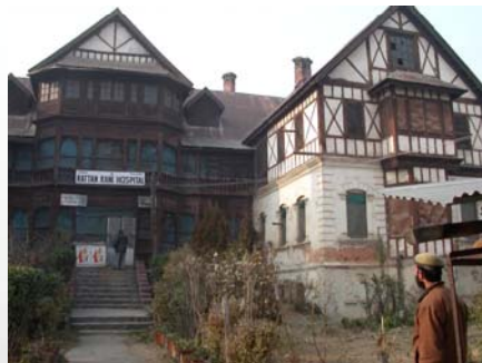
Dhajji Diwari construction in Srinagar area, Kashmir Patchwork of brick panels confined by timber members
