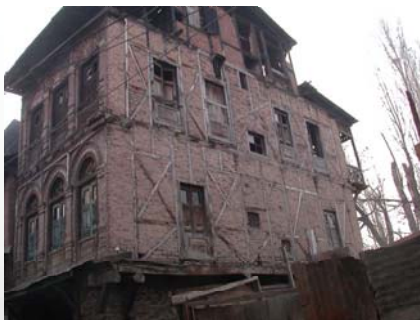
Dhajji Diwari construction in Srinagar area, Kashmir Patchwork of brick panels confined by timber members
