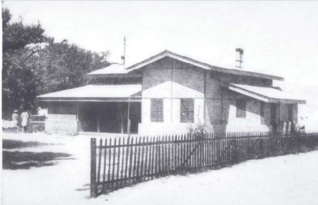
Six bungalows constructed by Kumar Brick walls braced with vertical and horizontal iron rails
