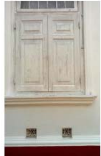
Air Inlet at the Ground Level
