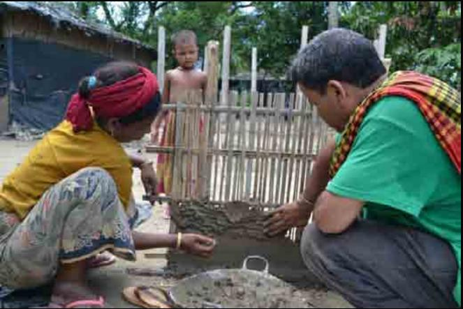
Wattle and daub wall with bamboo and cement stabilized soil Improving the local technique for stronger walls Horizontal and vertical cross-bracings make houses stronger
