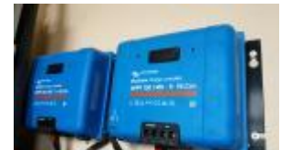
Solar charge controller at public health centre in Narayanganj
