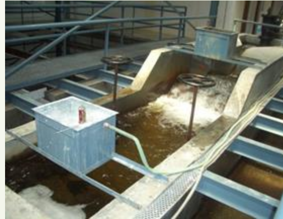
Flocculation Tank
