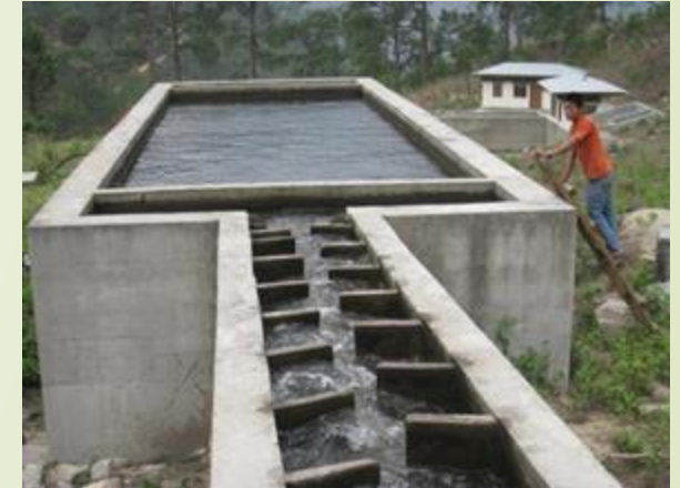
Sedimentation Tank
